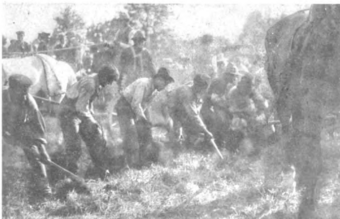
Workmen Getting Busy After the Speechmaking Ceased.
